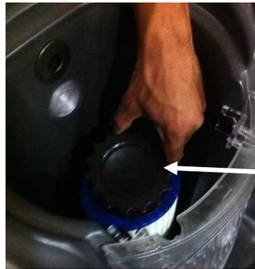
The spa's automatic surface skimmer filter is designed to remove floating debris and contaminants, such as body lotions, by drawing water through a specially formulated filter cartridge element. It is critical that this element be routinely cleaned.
